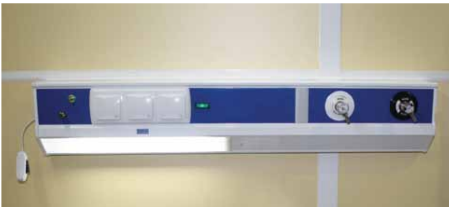
Wall ward consoles
